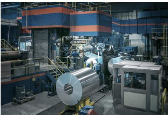
Cold rolling mill
